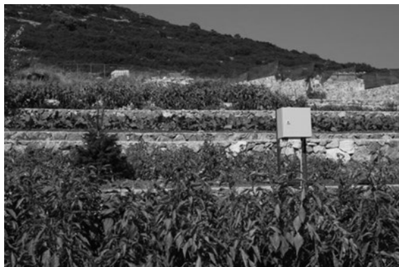
Figure 9.11 An installed QUHOMA AGRI node
