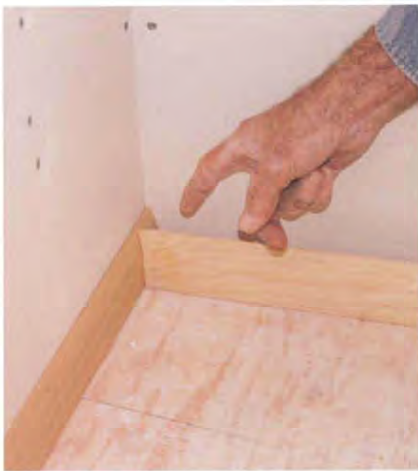
Coping trim at inside corners creates a tight-fitting joint.
