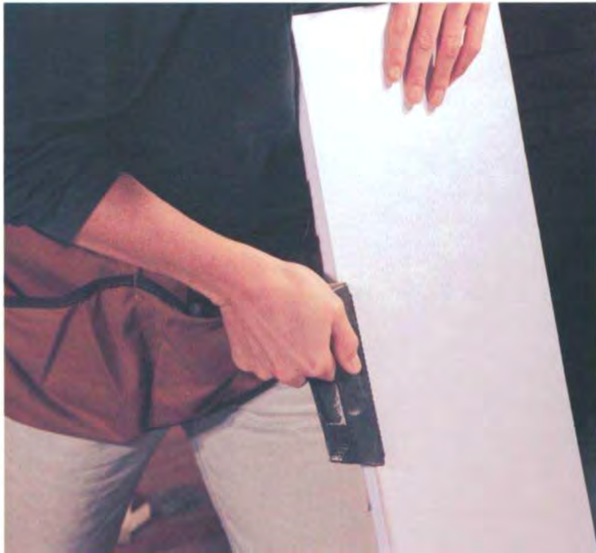
The Surform works well to trim a piece of drywall that doesn't quite fit.
