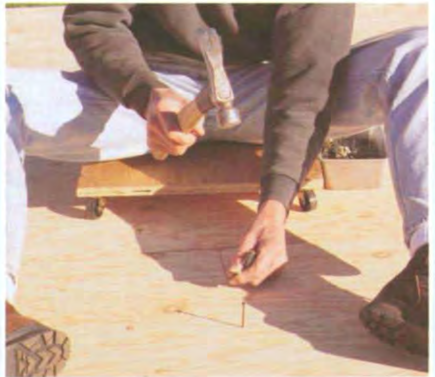
Sitting on a nail buggy makes it easier to nail floor sheathing. (Photo by Roe A. Osborn.)
