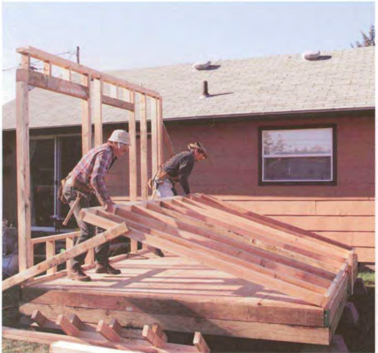
When raising a wall, keep your back straight and lift the wall to your waist using your legs. Then push the wall overhead with your arms and upper body until it is fully upright. (Photo by Roe A. Osborn.)
