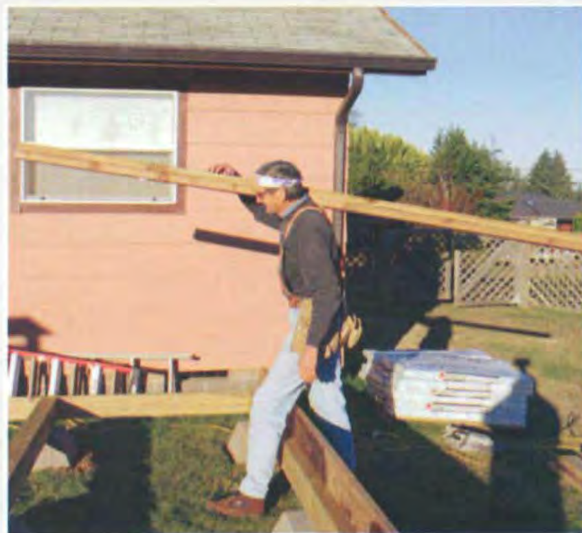
When carrying lumber around the job site, it's easier on your back if you balance it on your shoulders.
