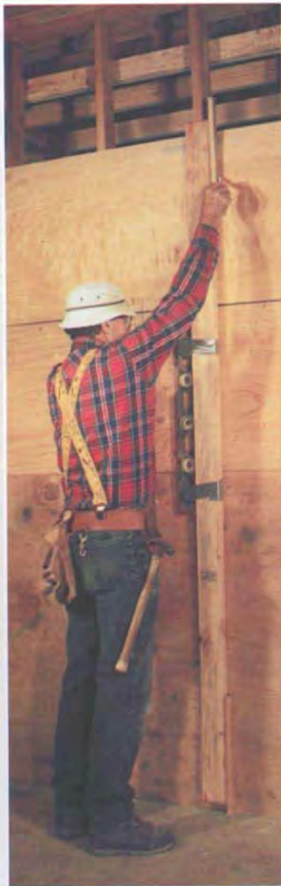
A plumbstick is useful for checking a wall for plumb. It is made of a straight 2x4 and a 2-ft. level.
