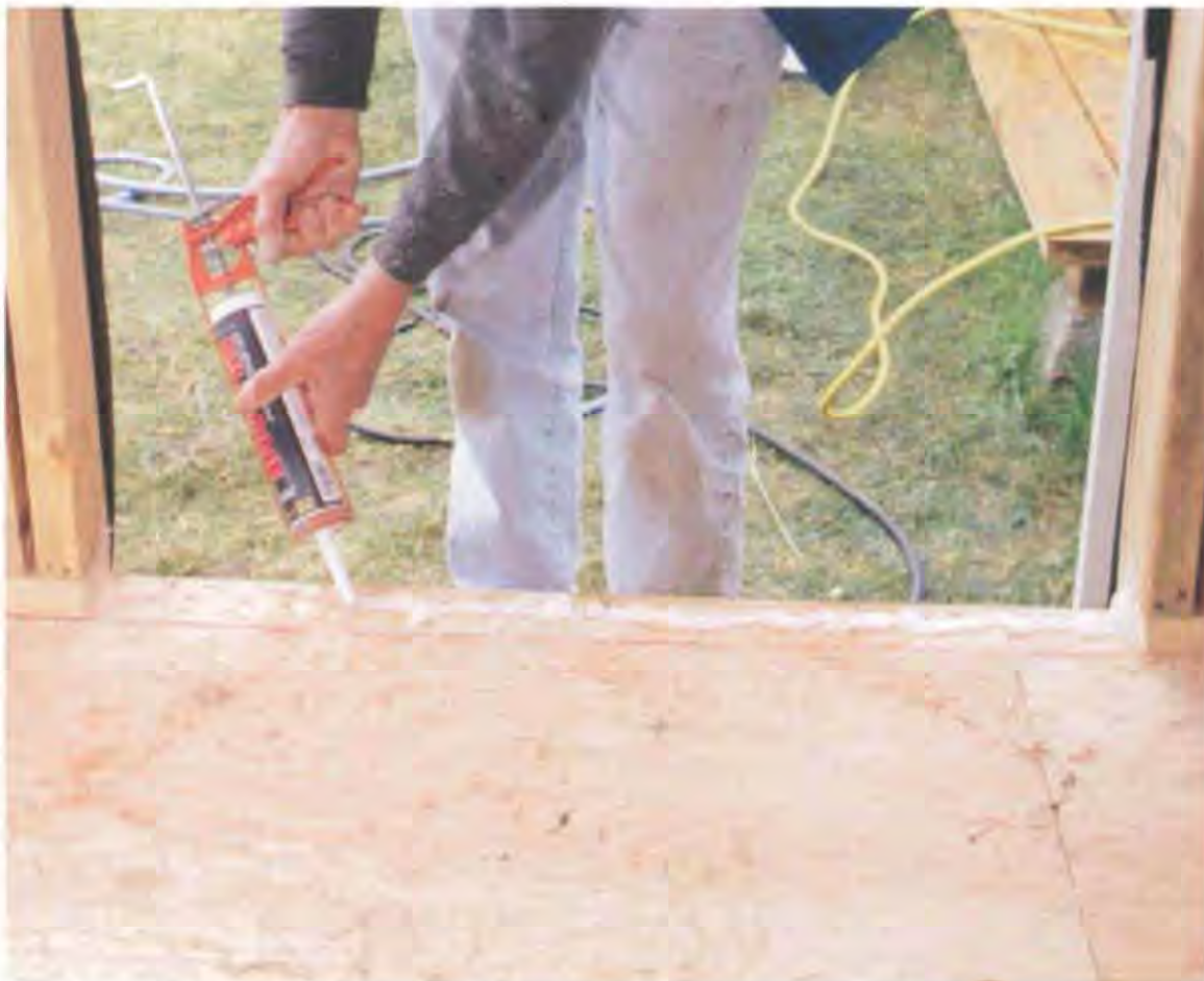
Wherever there's a danger of water getting into the house, such as under a door threshold, a bead of caulk can help seal the gap. (Photo by Roe A. Osborn.)
