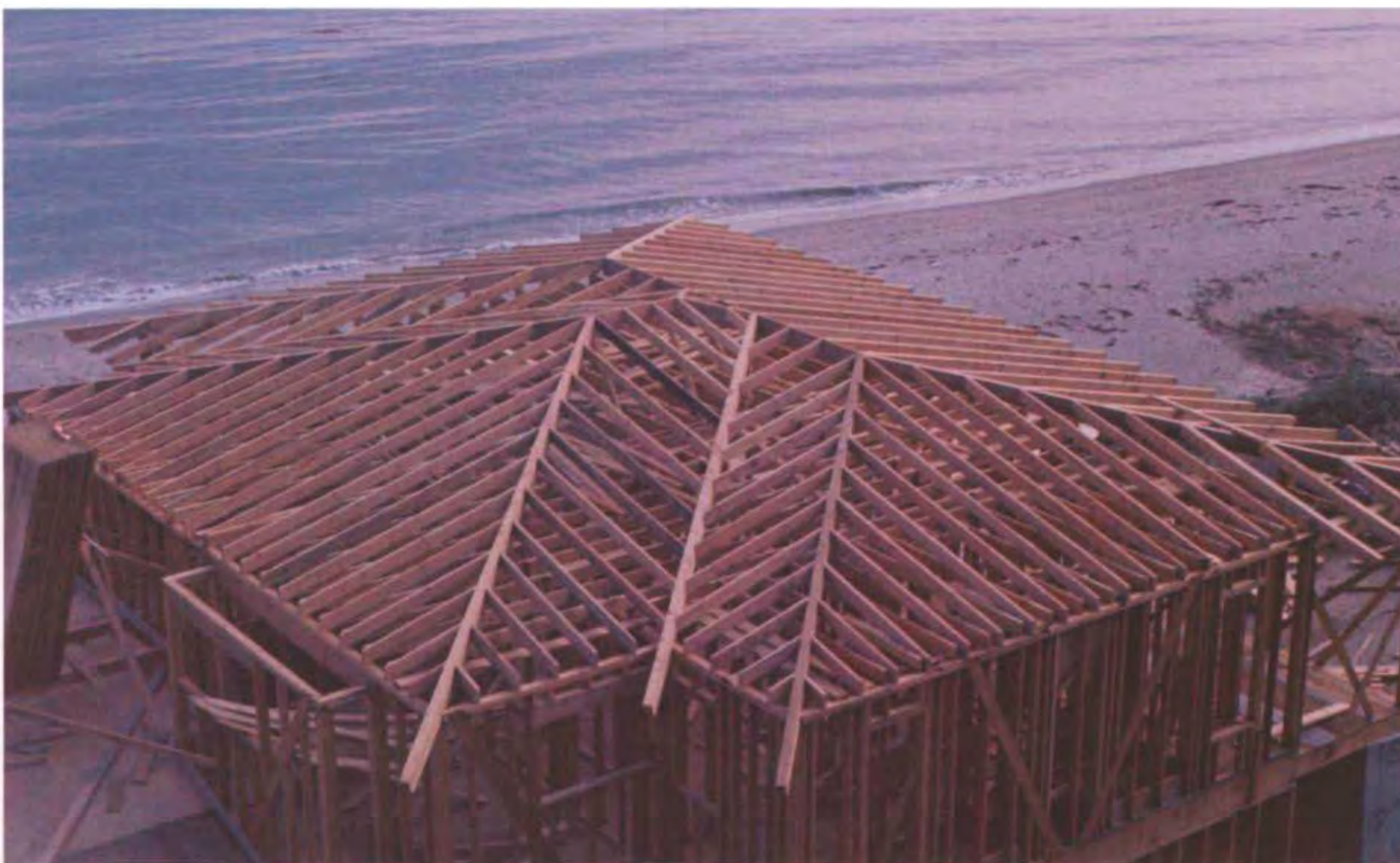
Conventional stick-built roofs can be framed as a simple gable or a complex roof with many different ridges, hips, and valleys. (Photo by Elmer Griggs.)
