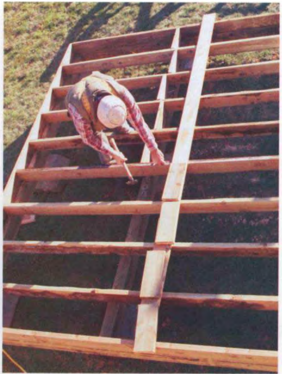
Floor joists form the platform, or floor, of the house and usually are spaced 16 in. or 24 in. on center.
