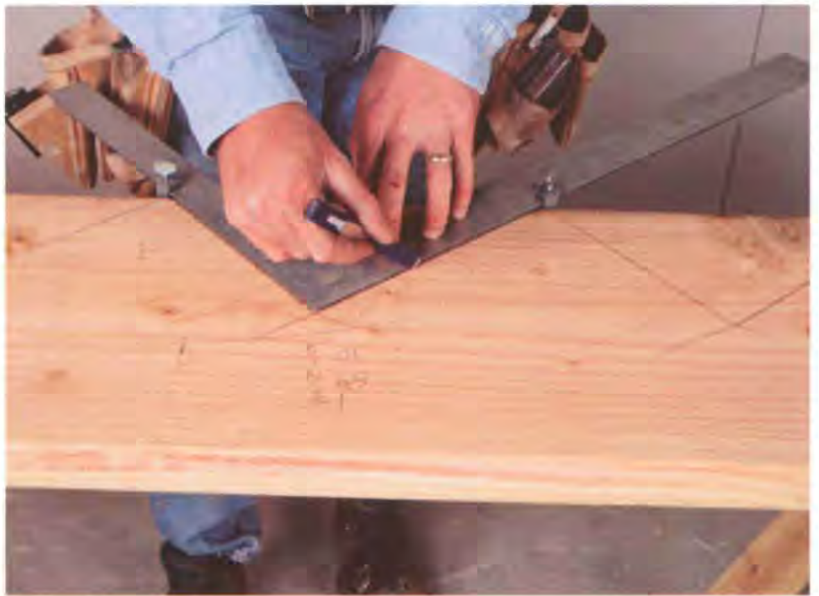
A simple set of stair gauges (small screw clamps that fix to the square) attached to the framing square makes it easier to lay out stair stringers accurately. (Photo by Roe A. Osborn.)
