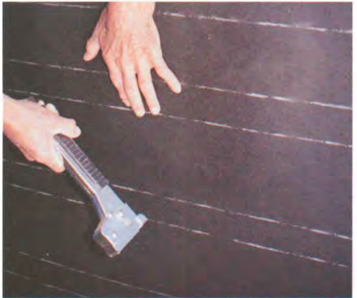
The hammer tacker makes short work of stapling down felt paper.
