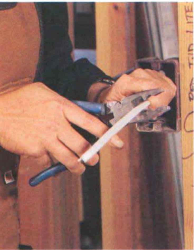
Side-cutting pliers are handy for cutting electrical wires.
