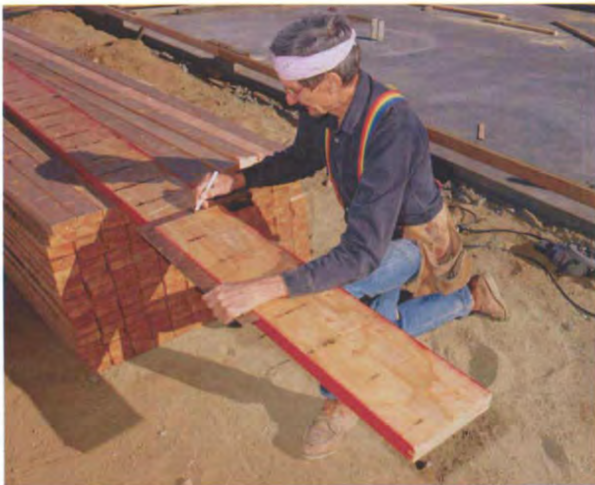
Construction-grade lumber used in house framing, such as the 2x12 I'm marking in this photo, must be structurally strong, but it's not necessarily free of knots. (Photo by Larry Hammerness.)
