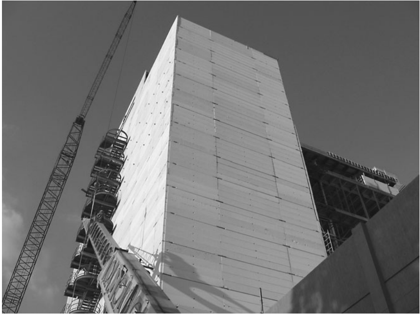
FIGURE 14.6 AAC cladding, Monterrey, Mexico. (Courtesy of Xella Mexicana.)
