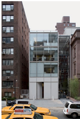
Glass is only used where new meets old or to provide light into spaces that do not house the collection. Photographer: Michel Denancé
