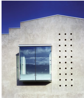
A window cutout in the existing wall underscores the surgical approach of the new intervention.
