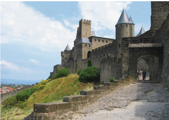
Mimicking the style of the surrounding architecture, Viollet-le-Duc added gate towers to the crumbling medieval city of Carcassonne, France, creating an inaccurate expression of the past.
