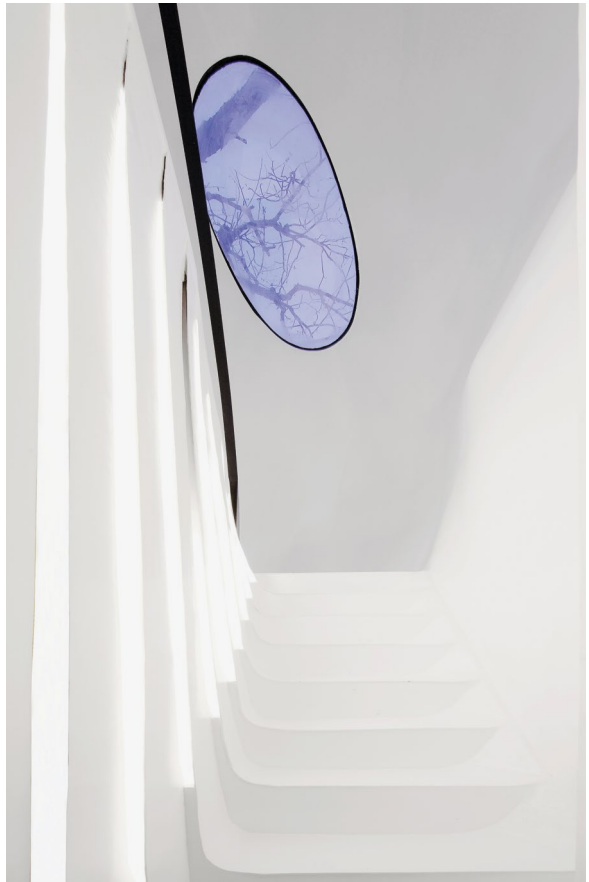
The staircase inside the bubble is cast into its skin.
