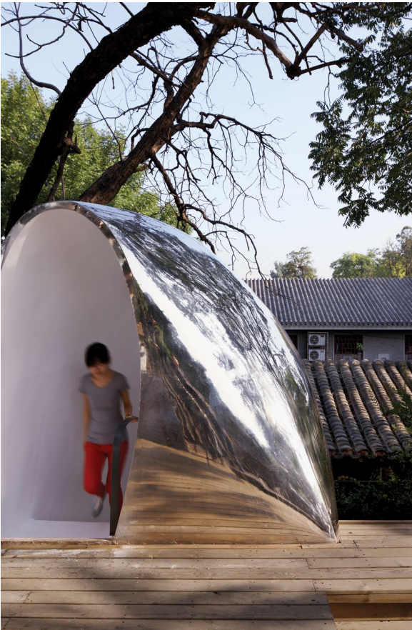
The entrance into the bubble is a simple displacement of the membrane's edge.
