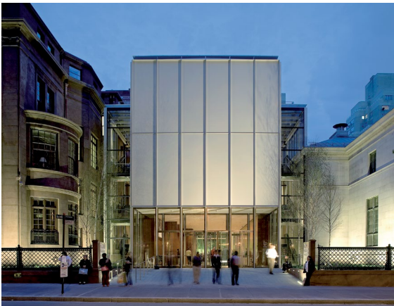
A successful design approach demonstrates visible interaction between new and old architectural styles. Addition to the Morgan Library, designed by Renzo Piano Building Workshop, New York, NY, 2006
