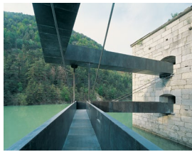
The bridge decks are channel-shaped steel gangways that are tied back to the structure with tension rods.
