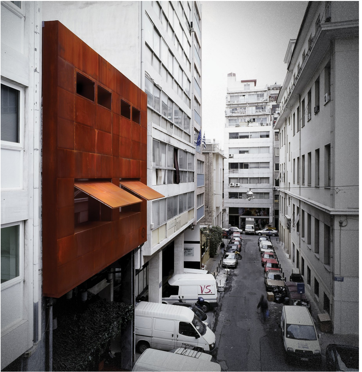
Openings in the giant steel door open and close in an array of configurations—in this case, slits and awnings.
