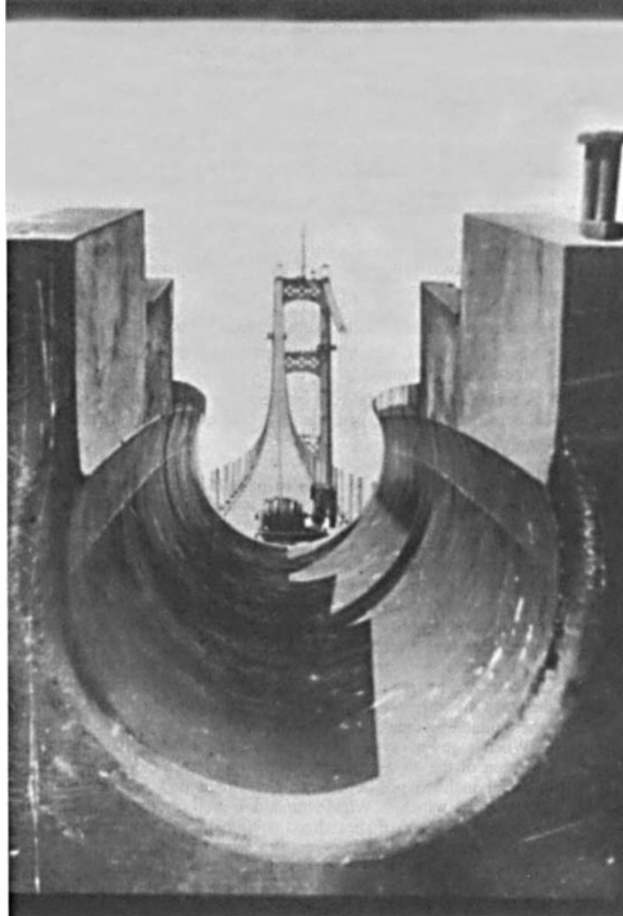
FIGURE 15.30 Pylon saddle.
