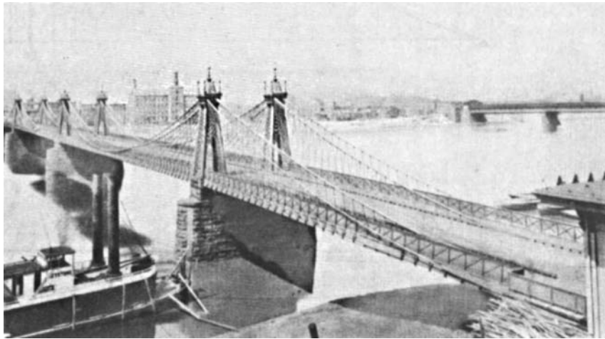
FIGURE 15.4 Old St. Clair Bridge, Pittsburgh.
