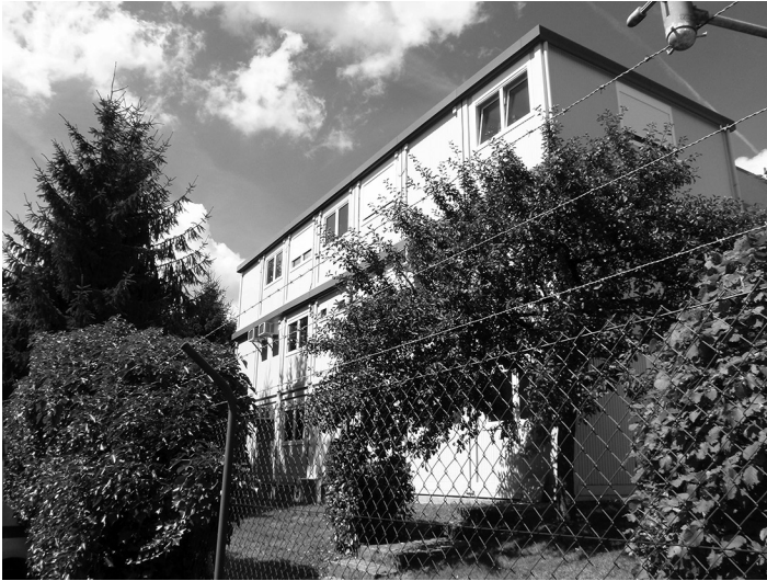
FIGURE 2.8 Container office War Room.
