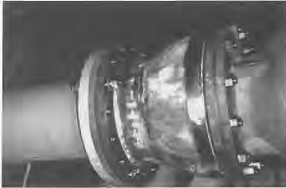
Figure 7.22 Application of an isolating plate and isolating volts to a seawater pump
