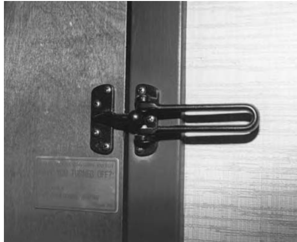
Figure 14-4 Locking device that replaces door chains at the Los Angeles Airport Marriott Hotel. Notice the lock in the unlocked position. When the lever attached to the door frame (right) is thrown across the ball attached to the door (left), opening the door will catch the ball up in the track slot, allowing the door to be opened only three inches. (Photo courtesy of the Los Angeles Airport/Marriott Hotel.)
