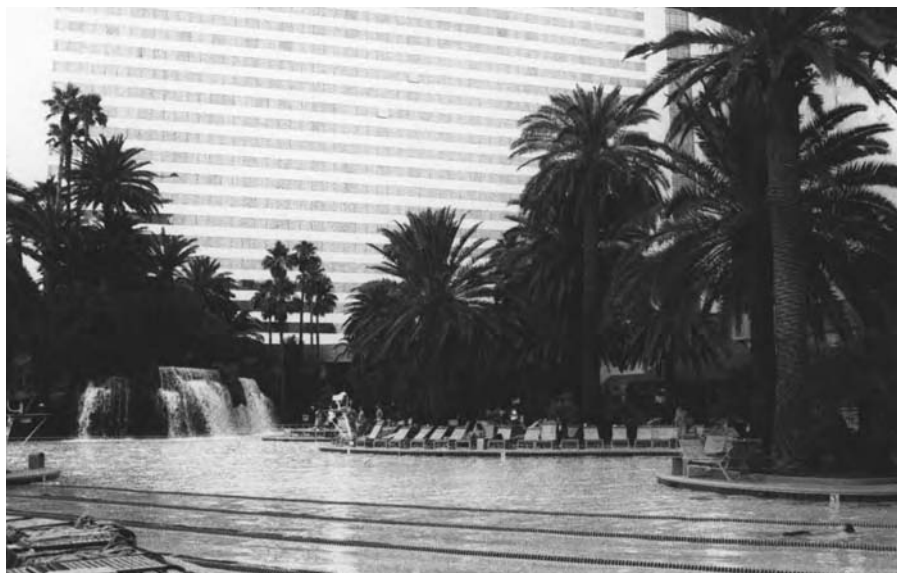
Figure 12-3 Mirage Resort main pool with hotel and waterfall in the background. The pool has a water surface area of 17,780 feet, 486,000 gallons of water, 1,033 feet of perimeter, 53 bottom returns, 35 inlet jets, 46 skimmers, and 6 drain covers that are 2 feet by 56 feet in length. There are also 555 feet of expansion joints built into the pool. Notice the three lap lines in the foreground. (Photo taken with permission of MGM Mirage.)
