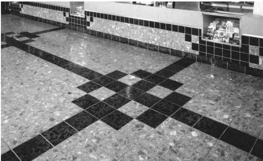
Figure 5-9 Agglomerate marble, a fabricated marble composed of natural marble stones blended with polyester resins, from Dal Tile Corporation. (Used with permission of Jacqueline & Associates, Las Vegas.)
