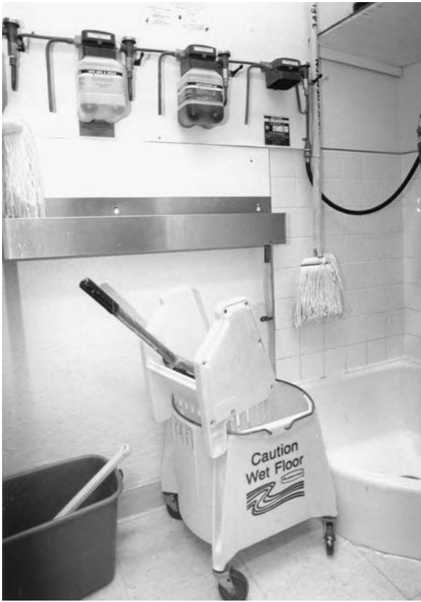
Figure 10-45 Another chemical mixing station located near a mop sink, in a satellite storeroom, allowing users easy access. Note the labeling of containers, required by Hazardous Communications Laws (HazComm). Information regarding hazards connected with a product must be clearly specified on the container. Products in smaller containers carry the same precautions as the container from which the product was drawn. (Photo courtesy of MGM Mirage.)
