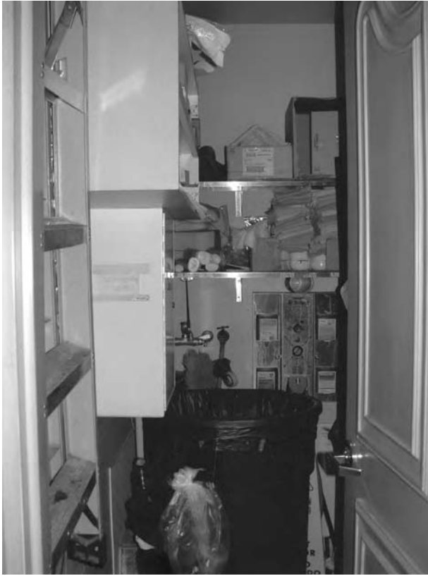
Figure 11-11 A typical public area utility closet at the Bellagio. Note the chemical mixing station at the rear of the closet. (Photo courtesy of Bellagio, Las Vegas, an MGM Mirage property.)
